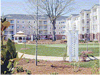
Photo: First Centrum Communities
